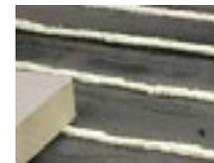
Insulation boards (**MW, EPS, PIR, PUR**) bonded with INSTA-STIK™ ROOFING STD applied with the **Hose&Wand applicator** (bead diameter of 20-25mm):
